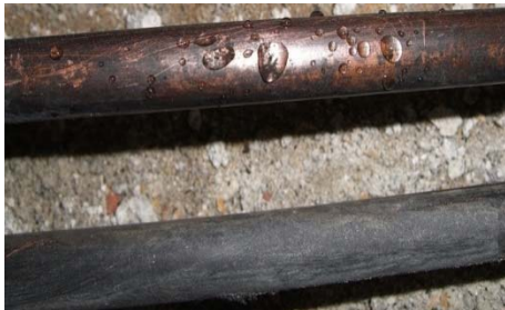
Damaged hydraulic hose pipe
